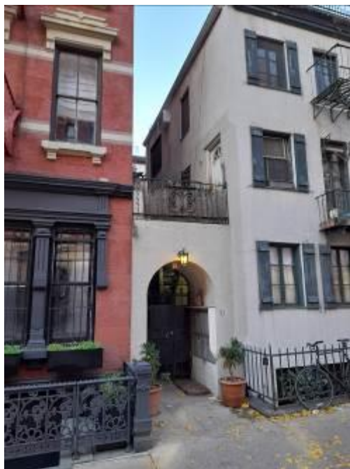
Fig. 1: 93 Perry Street, New York, NY 10014. This is the building that inspired Lovecraft’s short story
