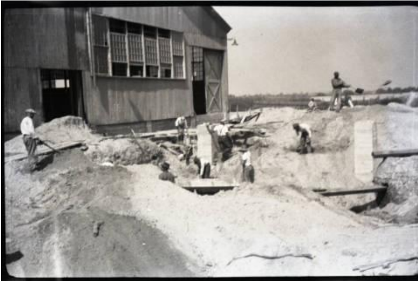
Fig. 8: Workers excavating a trench on the Panama Canal. MSS40_Box2_F9_86_001
