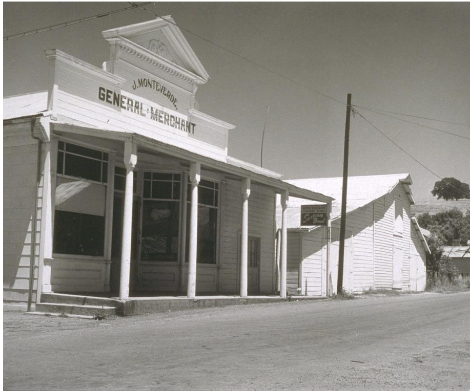
Fig. 1: Alma Lavenson, Monteverde [Monteverde's] Store, Sutter Creek, 1957. Bancroft Library, University of California, Berkeley
