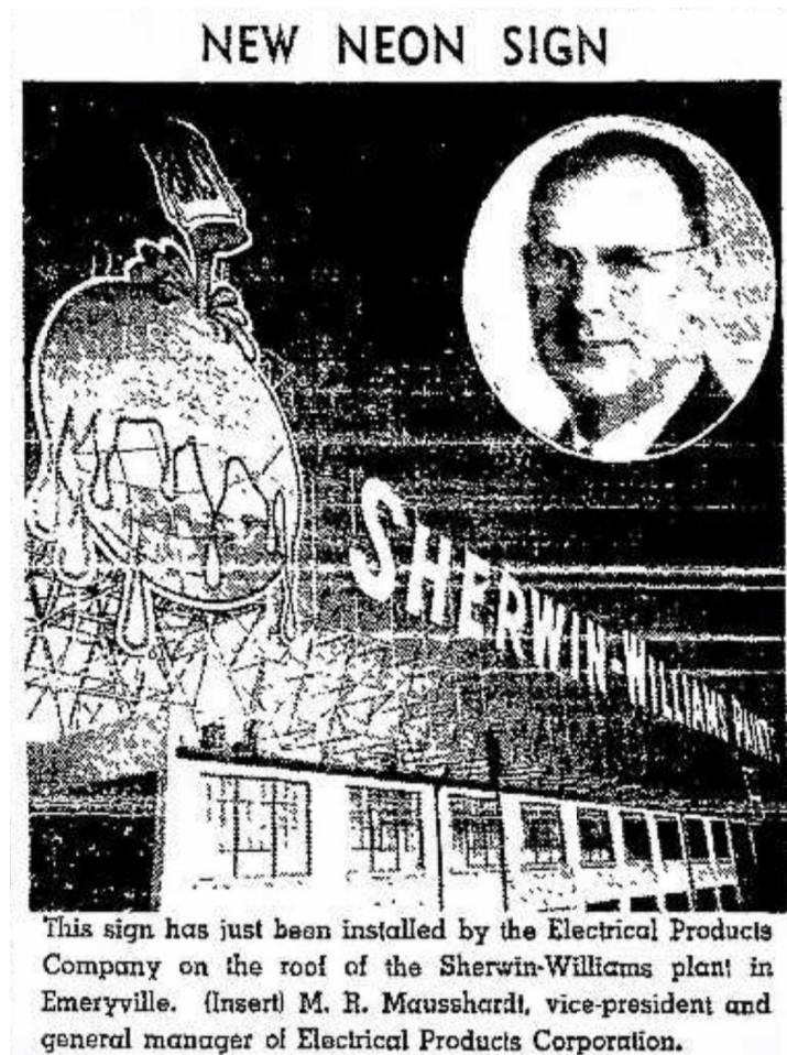
Fig. 1: Advertisement in the Oakland Tribune reporting the installation of the sign in Emeryville, April 2, 1939.
